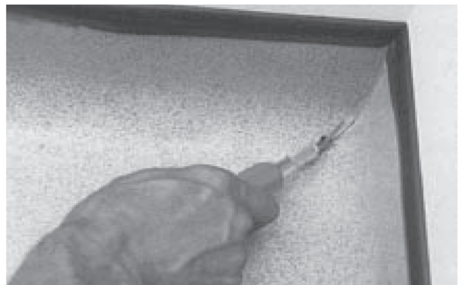
2. Trim the weldrod with the round router blade.
