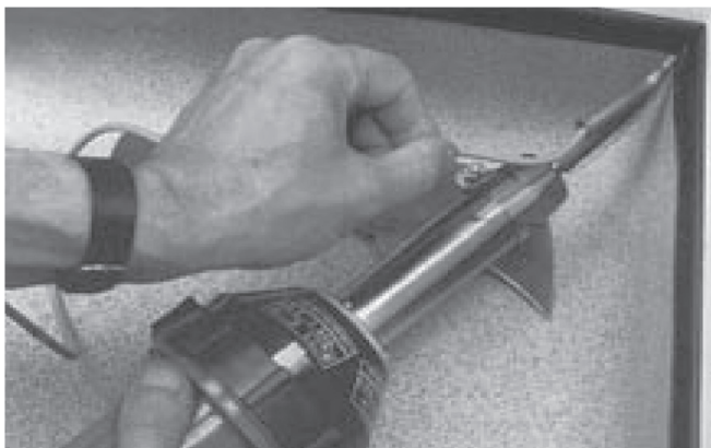
1. Groove the lower section of the joint, but not the upper. If the flooring has a PUR coating, all joints must be grooved prior to hot welding.
